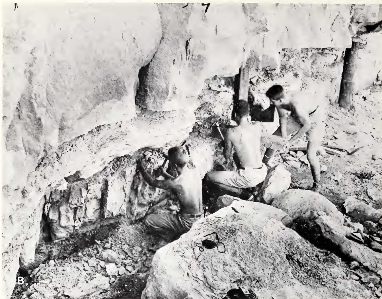
Fig. 2B. Installing timbers, early summer, 1954. Left to right, Wesley Williams, Richard Jones, William West.
